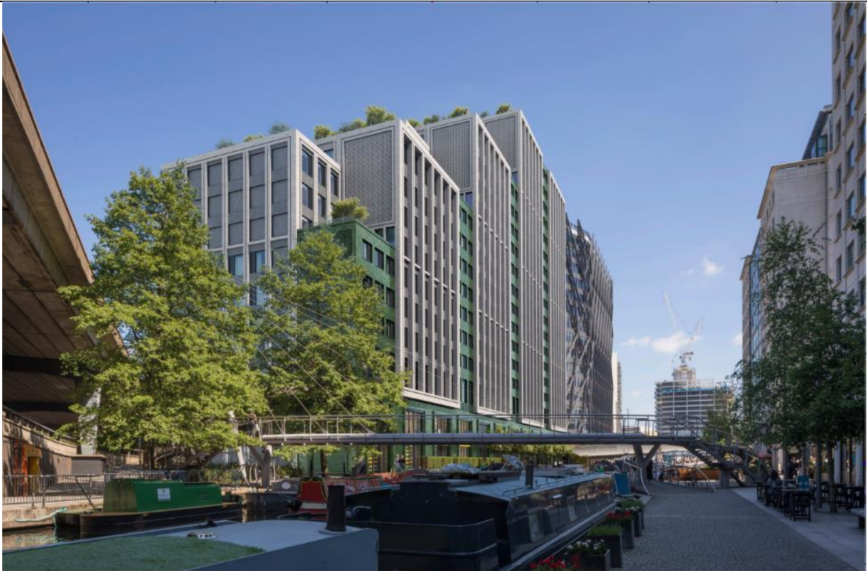
Verified view looking south east along canal
